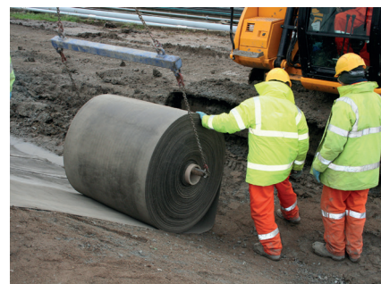
Concrete Canvas™ -betonikankaan levitys
