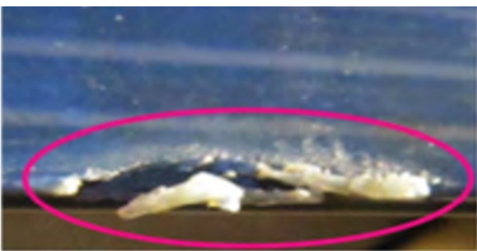
Figure 58: Discontinuity in surface smoothness due to CFRP damage
