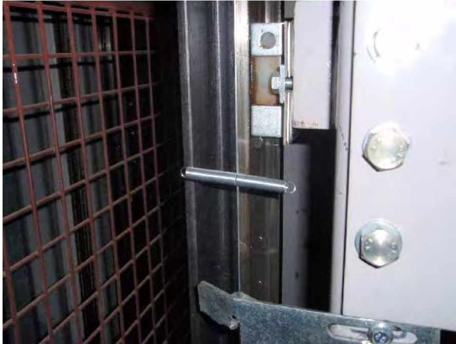
Figure 31: Shorting spring attached to string above top ring on CWT frame.
