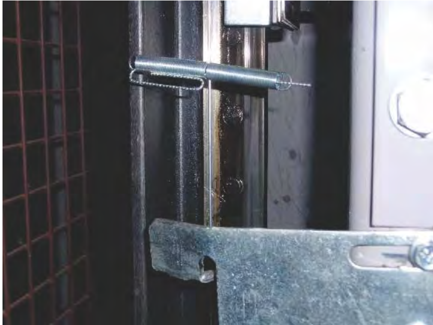
Figure 32: Steel wire inserted into shorting spring.
