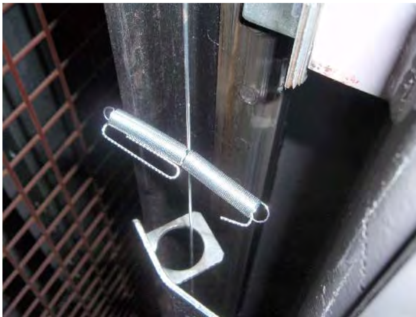
Figure 33: Steel wire is bent to ensure shorting spring cannot disengage from string during impact with CWT ring.
