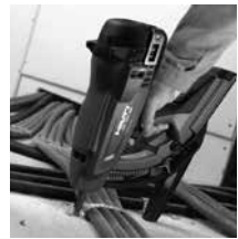
Conduits & pipes with metal or textile band
