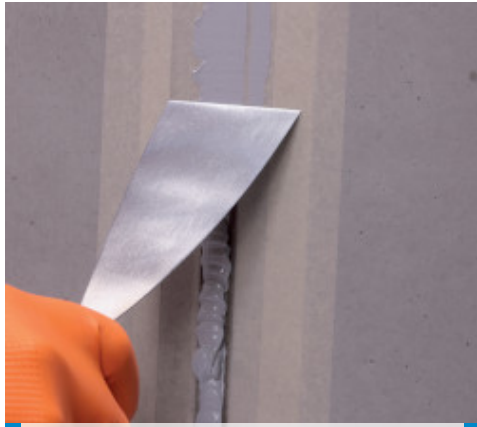
Smoothing over Mapeflex PU40
