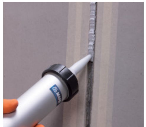
Application of Mapeflex PU40
