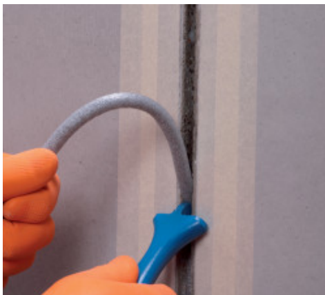
Inserting Mapefoam inside the joint
