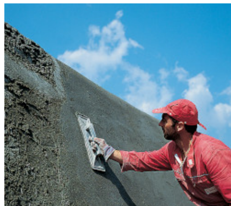
Finishing of MapegROUT T40
