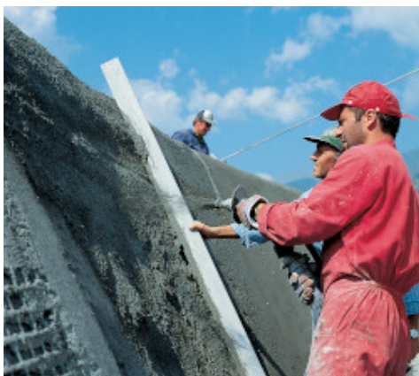
Spray application of MapegROUT T40
