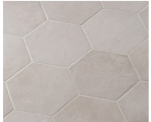
Floor grouted with Keracolor FF
