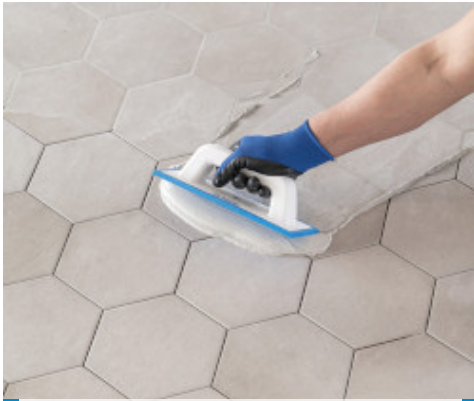
Application of Keracolor FF with MAPEI float
